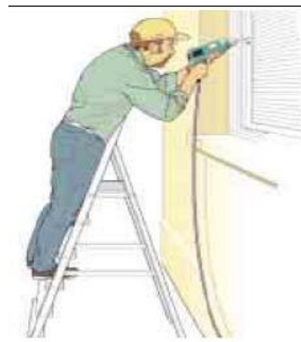
Correct – steps facing work activity
